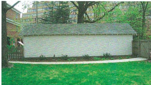
Side View of Garage (the garage is two car lengths long)
